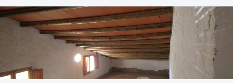
**4.1** The structures on site are in a state of good repair, though they will require refurbishment and updating. The roof is predominantly in excellent condition and some of it has brand new repairs; nonetheless, the owner has informed us about some historical woodworm damage that has already been addressed.
